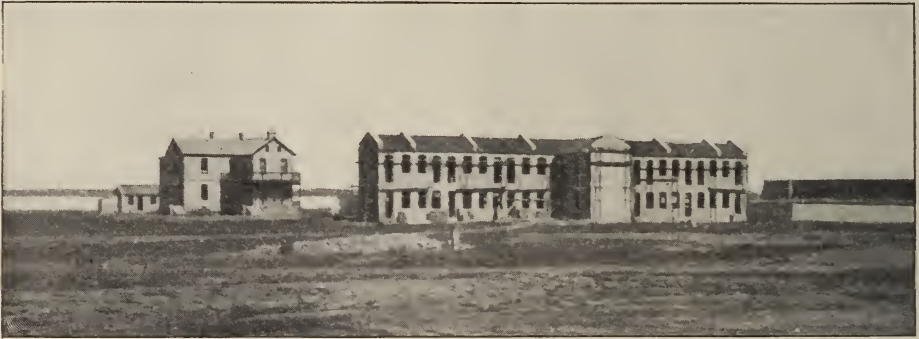
BOYS' SCHOOL DORMITORIES, MCCANN HOUSE, AND CITY WALL
